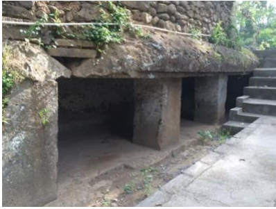
Figure 6: Cliff Temple Building
